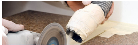
Marble Fitting Works
